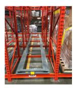
**Push Back** The pallets are loaded through an open aisle, one after the next. Each pallet pushes the previous one backward, using a subsequent pallet loading rail system.
